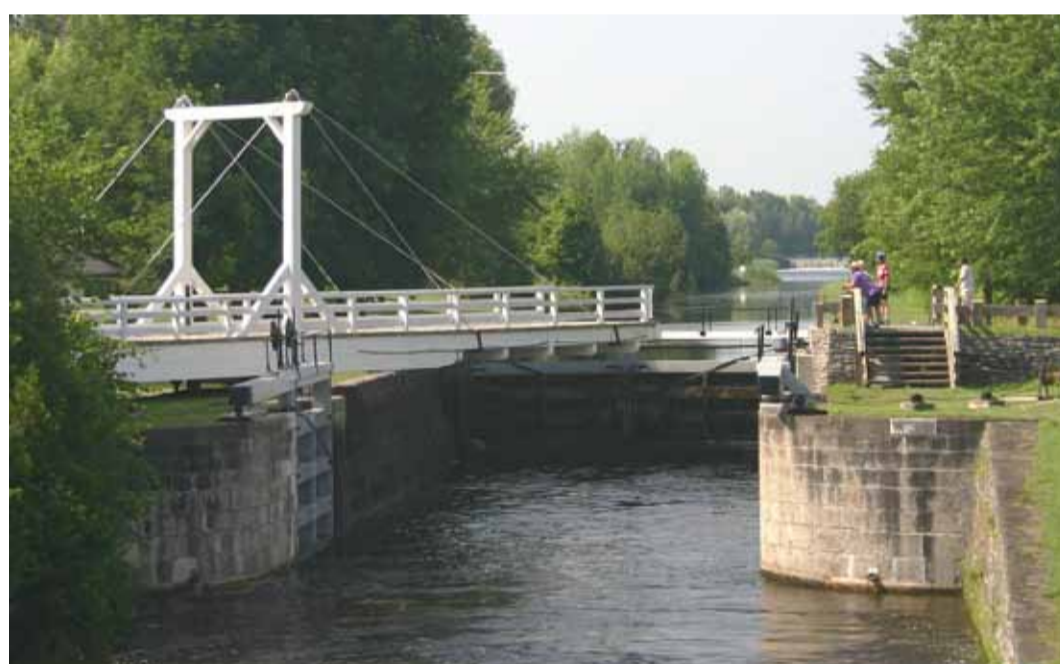
The king truss swing bridge and the lock at Nicholson's give a good idea of the type of engineering to be found on the waterway.
