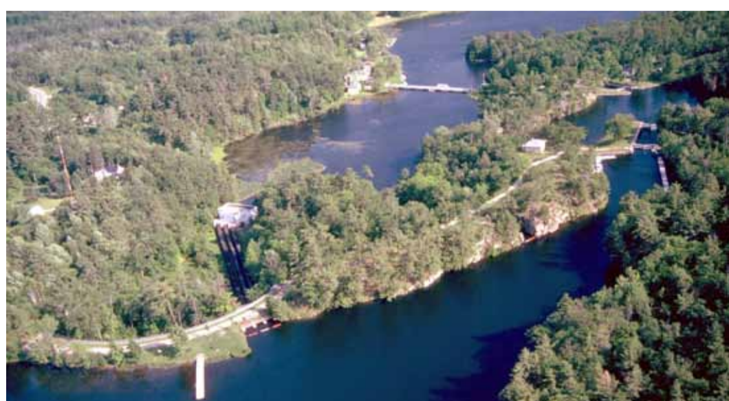
The hydro-electric station at Jones Falls.
