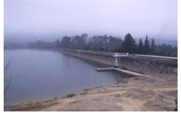
The reservoir at St Ferrol was the first such structure on a canal and is an important landmark in their development. By freeing canals from seasonal water supply variations, such reservoirs made the development of canals possible in places where water supply was restricted. Almost all English canals rely entirely upon reservoirs for their water.
