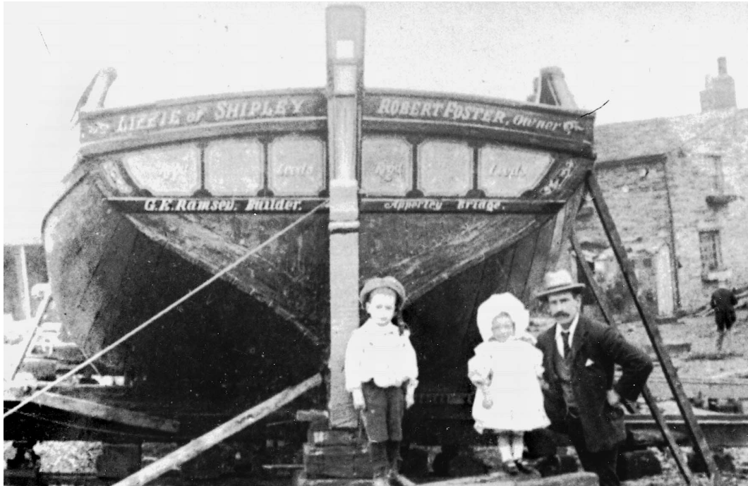
The Lizzie of Shipley on the slip at Apperley Bridge, near Bradford, around 1910. The transom is painted in the typical Yorkshire style, with simple panels surrounded by extensive lining. The boatbuilder, G E Ramsey, subsequently moved to Shipley.
