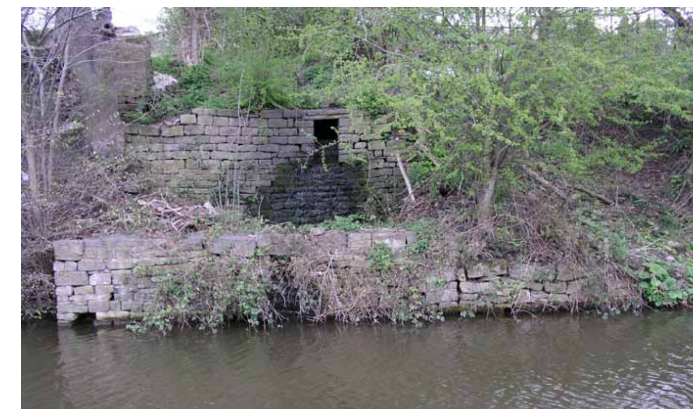
Land drainage provides some of the canal's water supply. Here a stream enters the canal at Dowley Gap via a 'stilling' bason to collect rubbish and silt.
