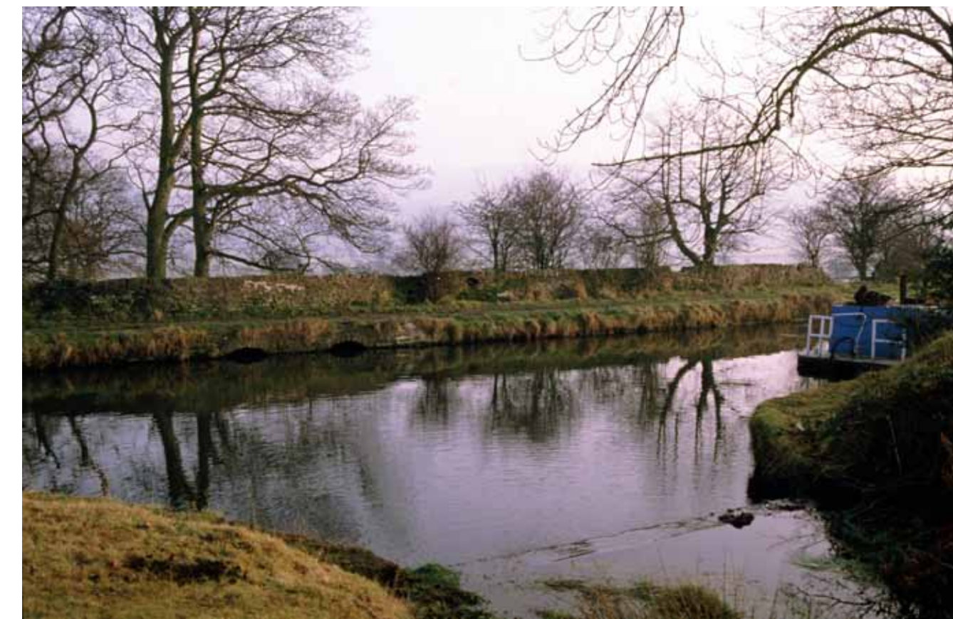
County Brook carries the water supply from White Moor Reservoir. It enters the canal on the right, with any excess water returning to the brook via the overflow under the towpath.
