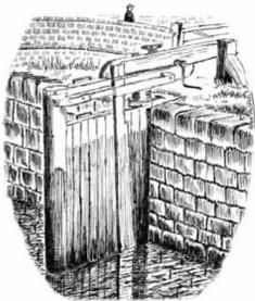
There were a wide variety of gate paddles on the Leeds & Liverpool Canal ground paddles. This one has a horizontal rack which pulls or pushes a long lever pivotted just above water level. This allows the paddle hole under water to be opened or closed.
