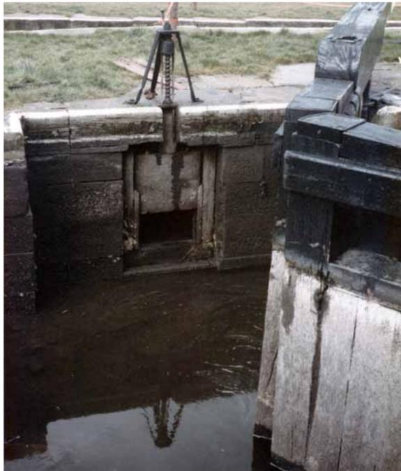
Two photos of upper lock gates which were taken when locks were being repaired. Both show ground paddles, but of different types. On the left is a 'box clough', where the paddle covering the drain hole is raised by a screw. This one is held in an iron frame, but usually they are in wooden boxes, as in the drawings above right.
