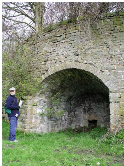
Around 15 canalside lime kilns still survive, such as the one on the left near Stockbridge. The canal is behind the kiln and out of sight at the top of the photo. Coal and limestone were brought here and loaded into the kiln at the top, at the side of the towpath. After burning, the lime could be removed through the square hole visible at the base of the kiln. Kilns were often located near streams so that the lime could be 'slaked' when hot, immediately after being removed from the kiln.
