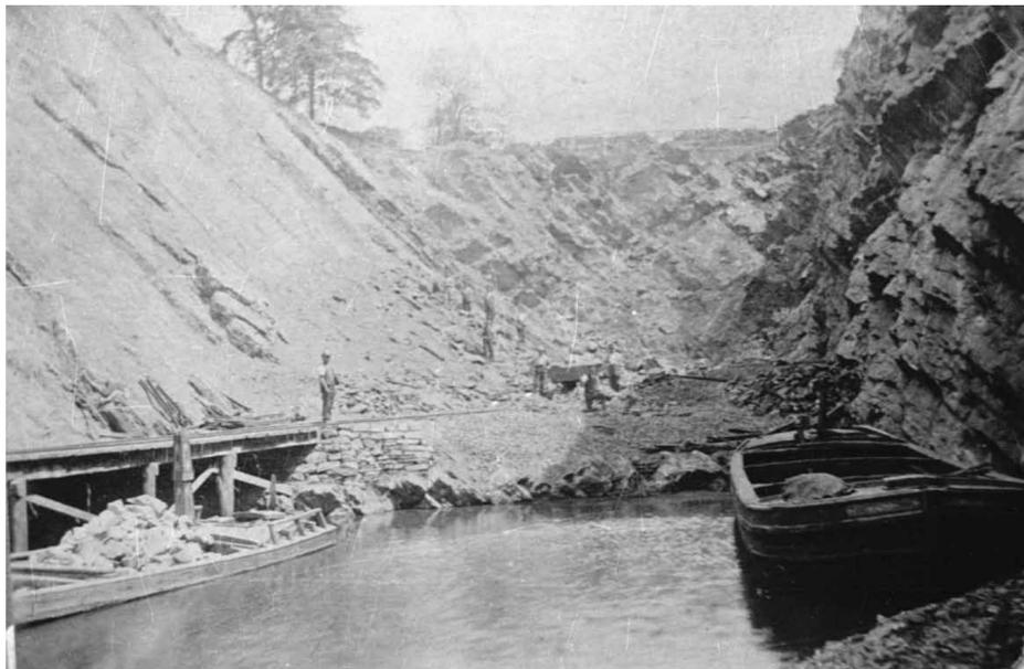
Rain Hall Quarry was at the end of a short branch canal which had two tunnels. Stone was loaded into boats virtually at the quarry face, as can be seen from this photo of circa 1895.
