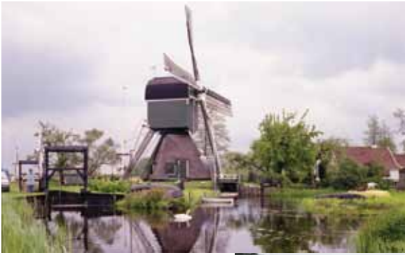
Left: The lock and windmill driven drainage pump at Tienhoven, near Utrecht. Lifting gates continued to be used on navigable drainage canals, where boat size was small.
