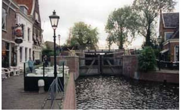
With variable water levels due to flooding or tidal action, gates often needed to hold back water in both directions. This led to two sets of gates, and the development of the chamber lock
