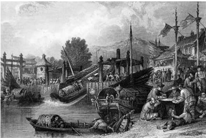
Left: By the time Europeans visited China regularly in the late 17<sup>th</sup> and 18<sup>th</sup> centuries, silt was a major problem for boats using the canal. Inclined planes replaced some locks, and simple flash locks using stop log gates were also used. These were much less likely to be affected by the increasing volumes of silt entering the canal from the Yellow River.
