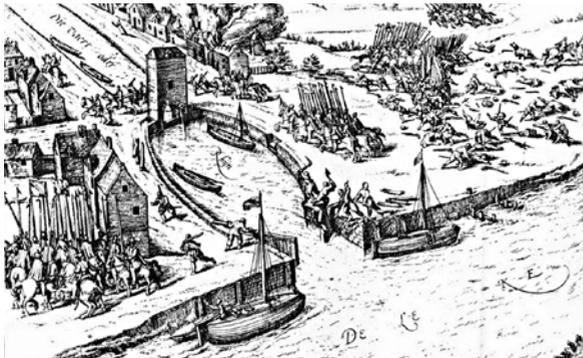
Above: The Kolksluis was the second lock at Spaarndam, and was built in 1290, rebuilt in 1571, and again in 1778. Originally it probably had lifting gates, with the mitre gates installed during subsequent rebuilding.
