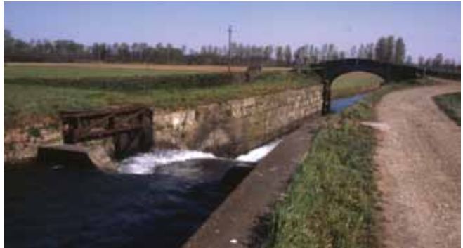
Above: A recent photo of a lock on the Canal de Bereguardo. The canal is still used for irrigation, and the locks have been rebuilt since chamber locks were first used here in 1458.
