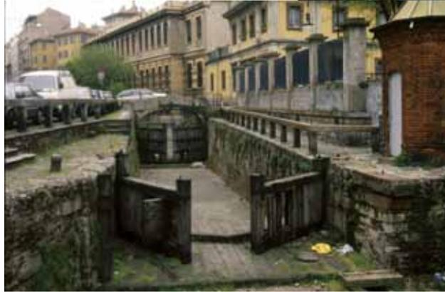
Left: One of the locks Leonardo da Vinci built in the centre of Milan. It has been restored using his drawings as a guide, with mitre gates and the paddles which rotate on a vertical axis.
